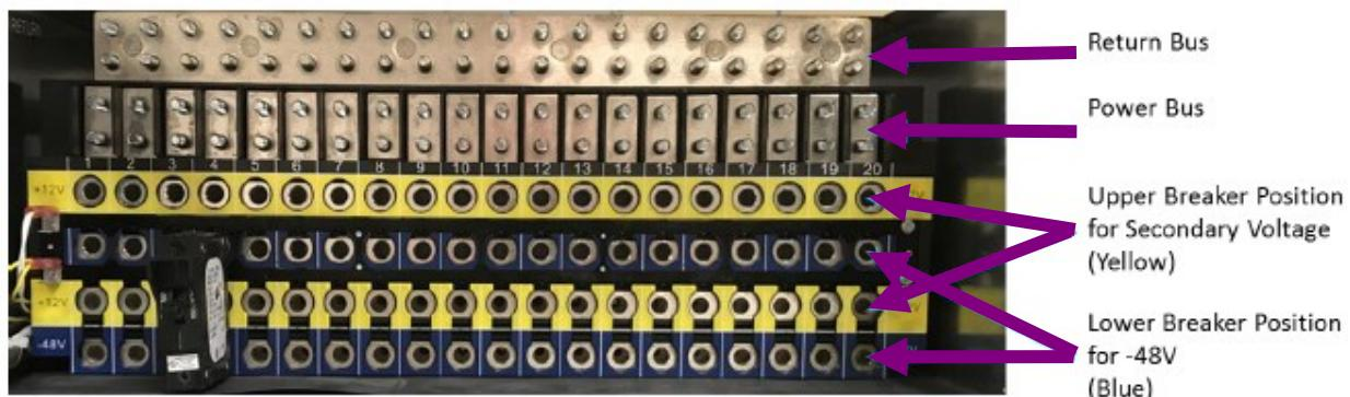
Distribution panels are each equipped with 20 (19" panel) or 26 (23" panel) bullet-style distribution positions. Each position is selectable between Primary or Secondary (Converter) Voltage outputs.
